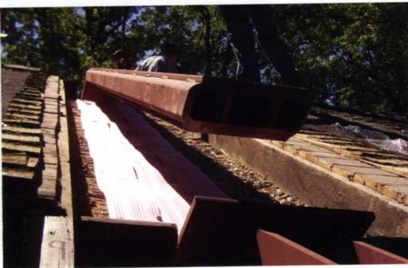
Precision placement of the roof beam to tie into vertical members on north and south sides of the house.
