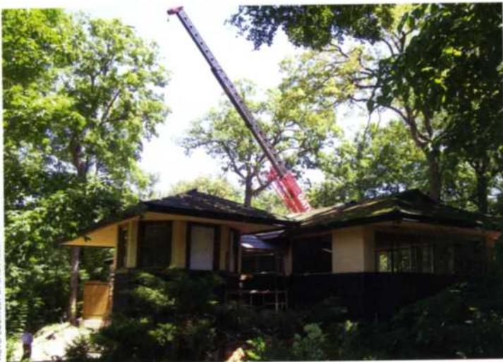
Crane inserting the steel roof beam in 2008.
