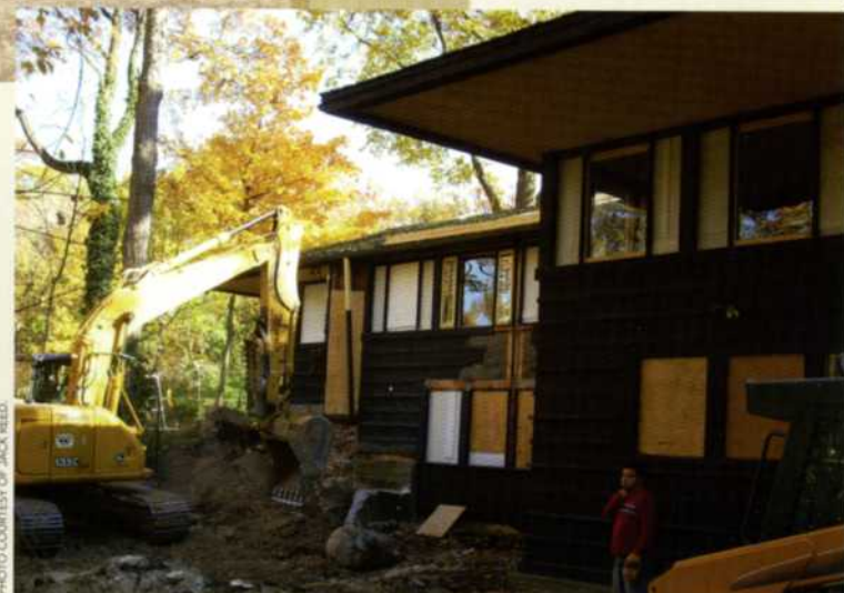
Removal of non-original stairway to restore original facade.
