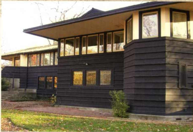
Northwest view of the Glasner House in 2004 with patio and stairway.
