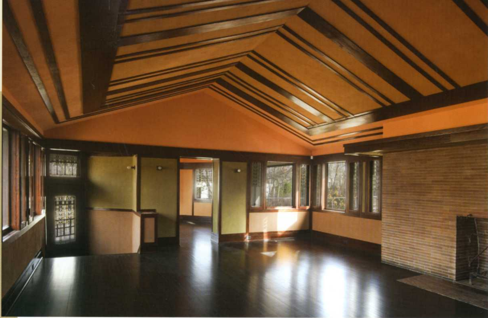
Living room after restoration, with steel beams in place, refinished original oak floor and original color palette for walls.
