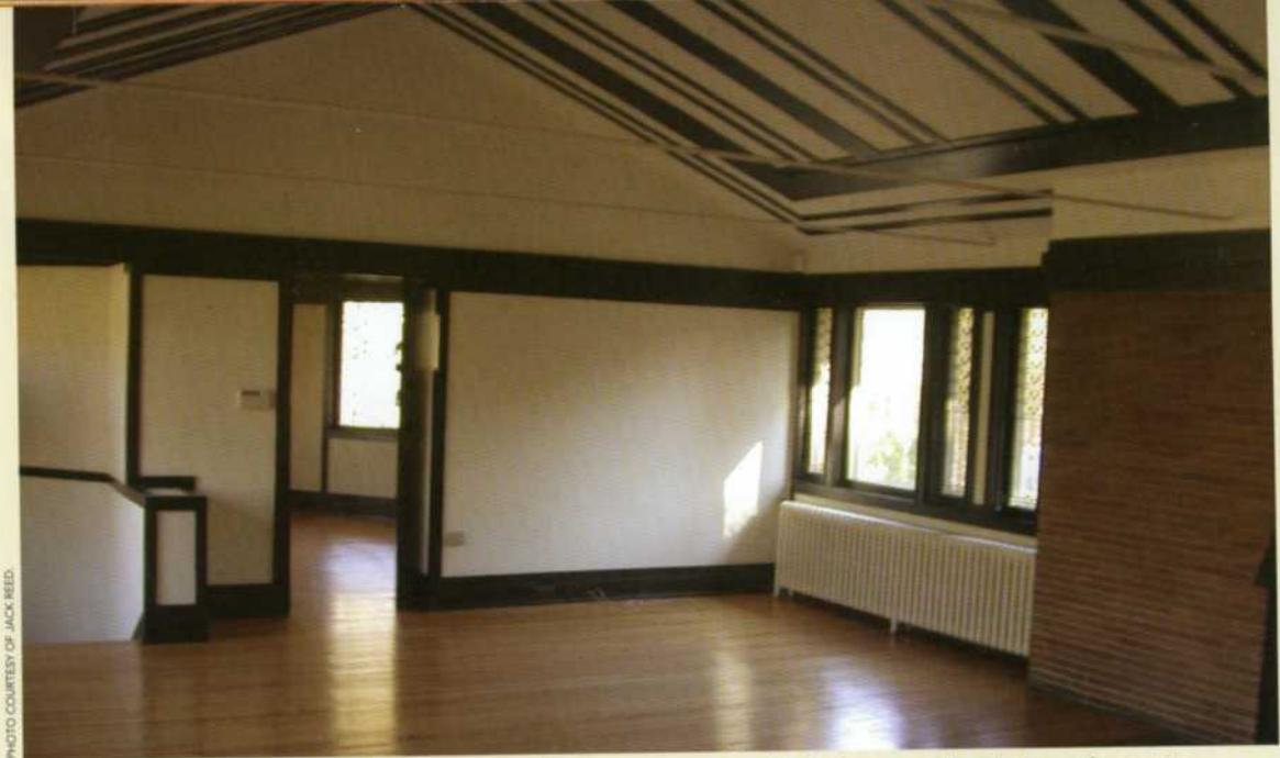
Living room in 2004, modified over the years to remove one set of windows, and with tie-rods across the room to keep the walls from spreading apart.
